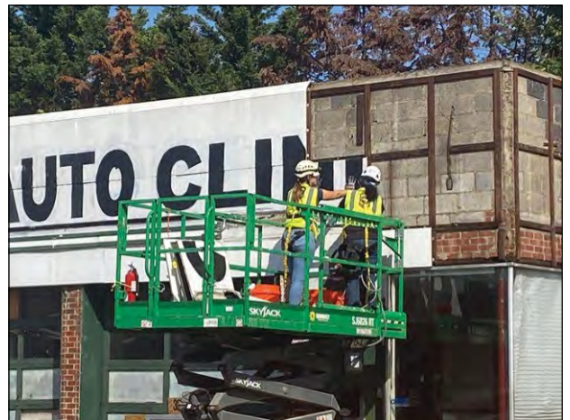
Dismantling of the Joyce Motors panels for restoration. Photo by Toby McIntosh.
